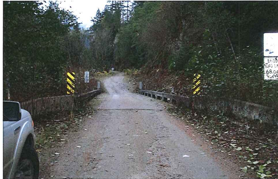
CK2143 Approach Left Bank
