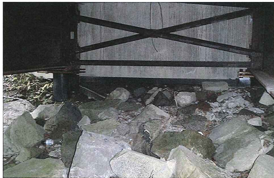
CK2143 Abutment Right Bank
