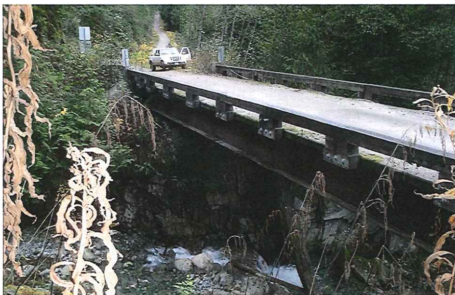
CK2143 Crossing Upstream
