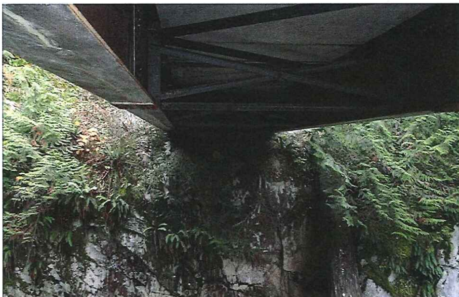
CK2143 Abutment Left Bank
