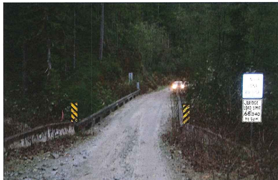
CK2143 Approach Right Bank
